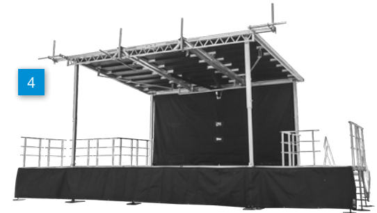
Install stairs, guardrails and add accessories.
